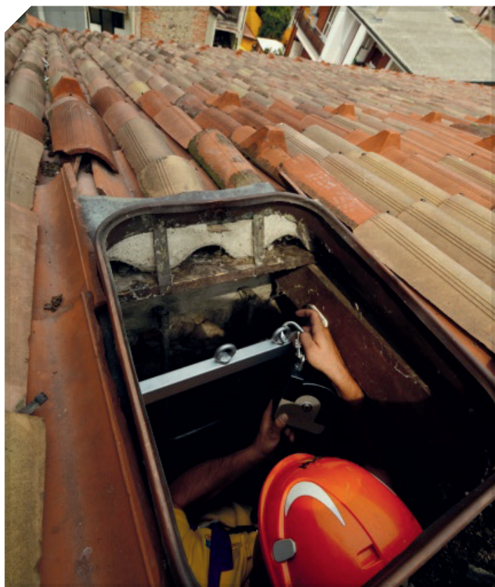
Fixing to the dormer, for roof work
